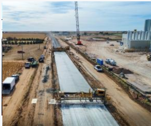
County Road 217 under construction
